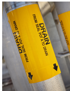
PIPE MARKERS PLACED IN HVAC INSTALLATION
